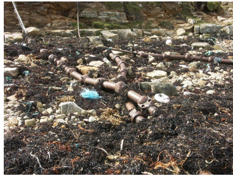
Submarine communication cables crossing the Scottish shore at Scad Head on Hoy, Orkney . By The original uploader was Jmb at English Wikipedia. - Transferred from en.wikipedia to Commons., CC BY 2.5, https://commons.wikimedia.org/w/index.php?curid=2111378
